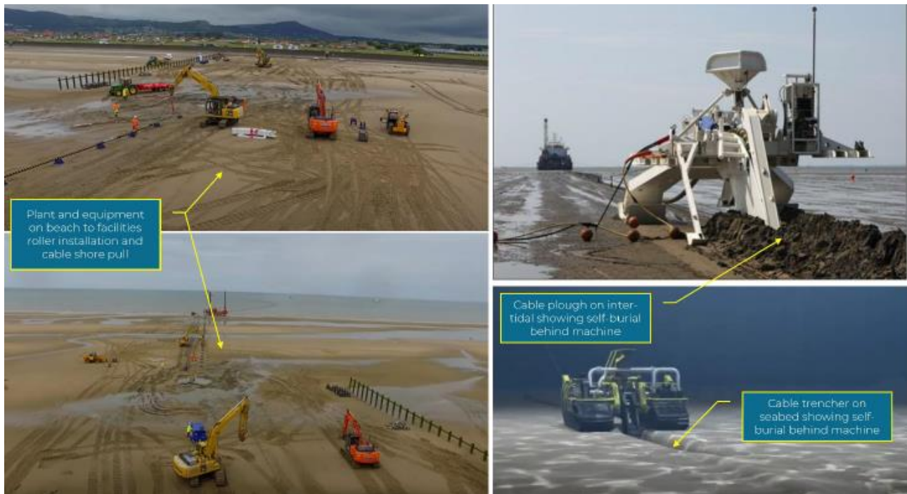
Figure 4.3: Typical plant and equipment for cable installation across inter-tidal like the offshore wind farm cables historically installed between Prestatyn and Rhyl.
